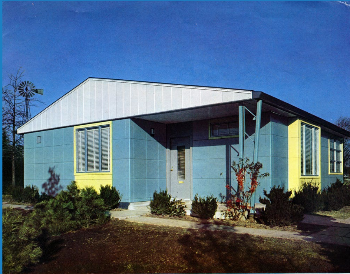
All metal Lustron House – 1949: 10 in Kansas City
