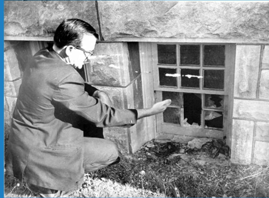
Damage from 1968 Riots
